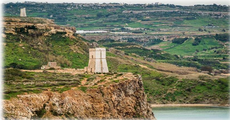
Two coastal watch towers. https://travelpast50.com/watchtower-golden-bay-malta/
